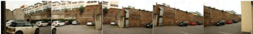
35 Commercial Street facing south-east (north wall)
