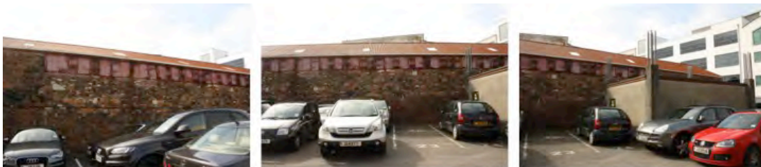
29 Commercial Street facing south-east (north wall)
