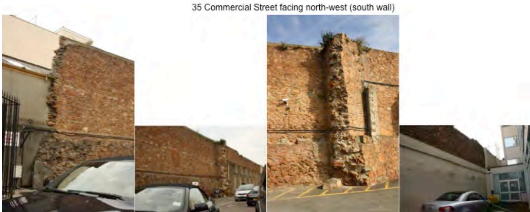
35 Commercial Street facing north-west (south wall)
